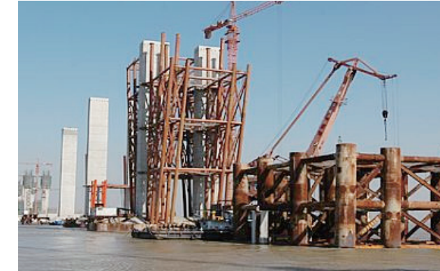
苏通大桥 Sutong bridge
