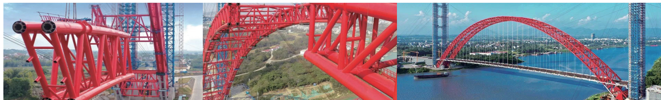
平南三桥 Pingnan Third Bridge
